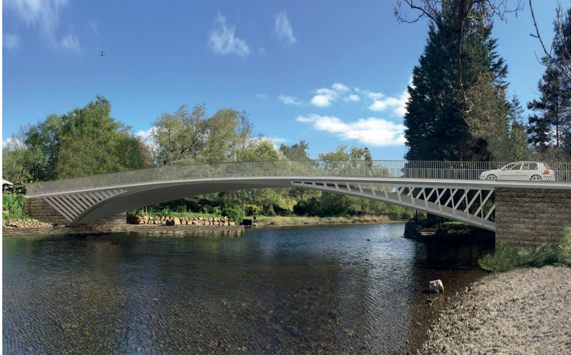
Design consensus The form of the new Pooley Bridge was chosen after extensive consultation with the local community
