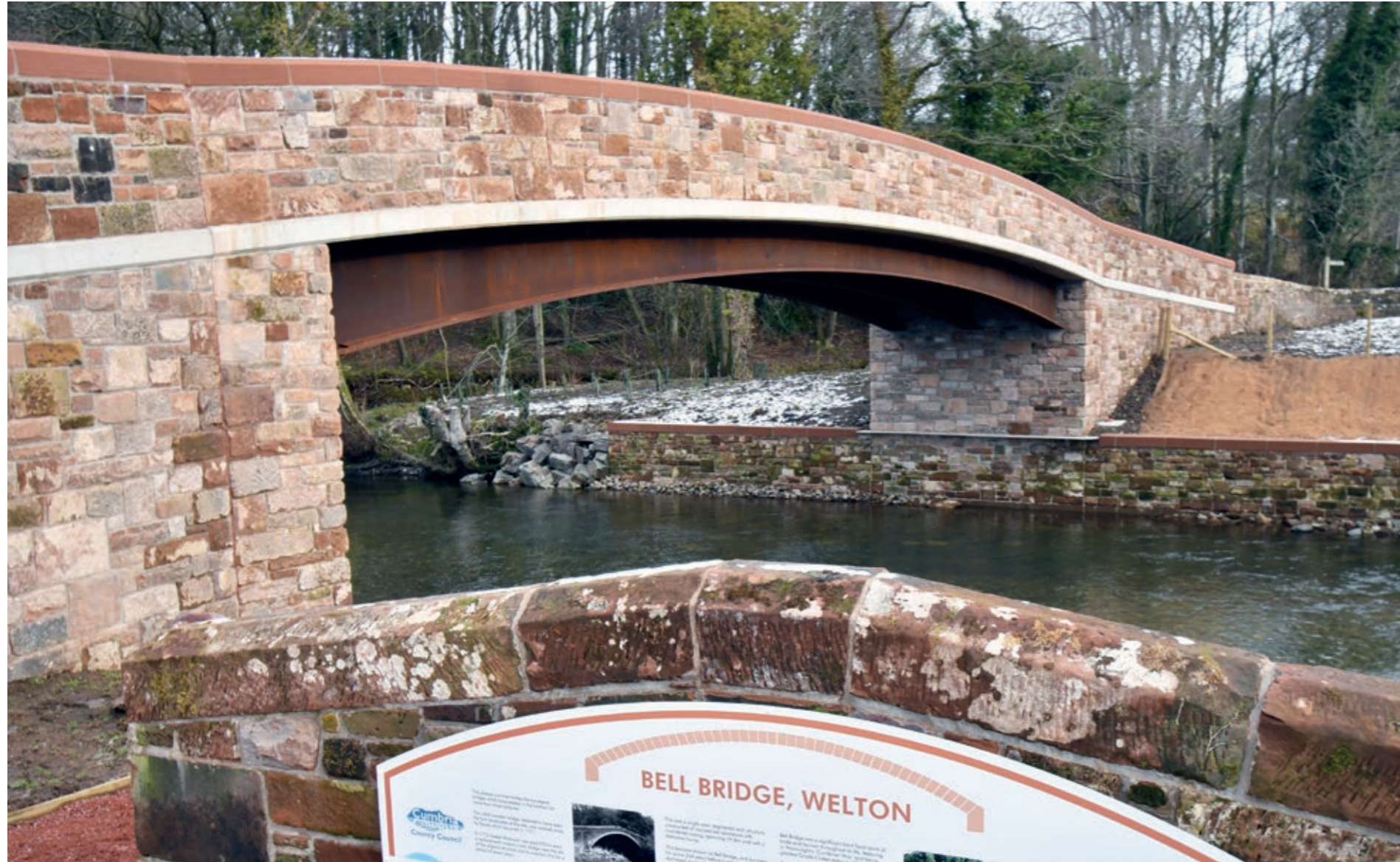
Resilient design The new Bell Bridge has a designed working life of 120+ years
