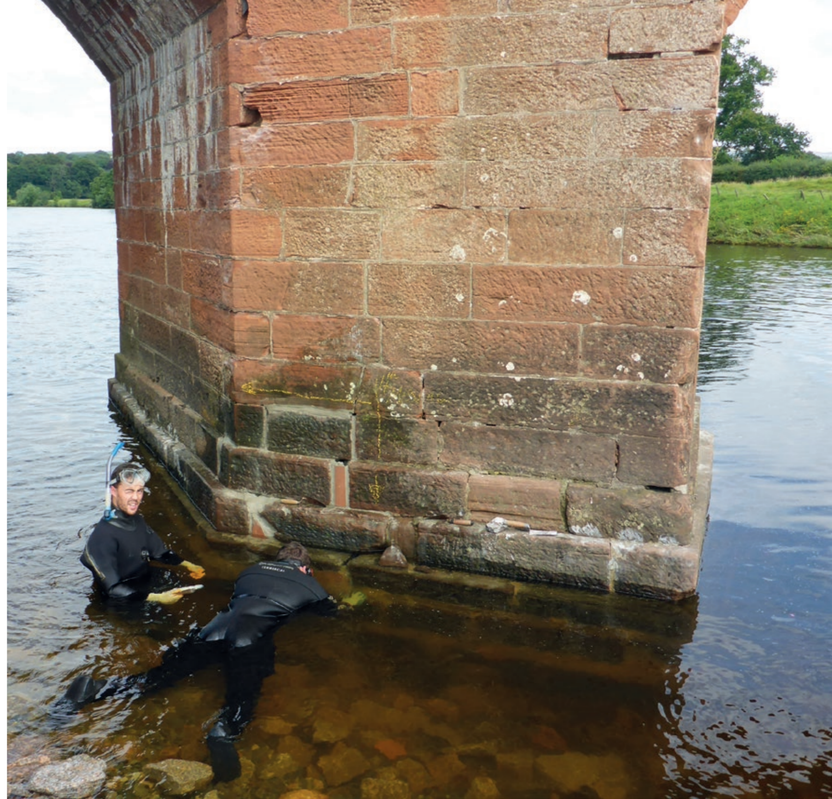
Structural inspection Engineers checking for scouring damage at Lazonby Bridge
